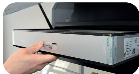
Fig. 49: Remove the HEPA filter
